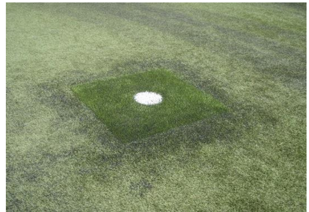
Photo 31: Replacement penalty spot due to excessive wear
