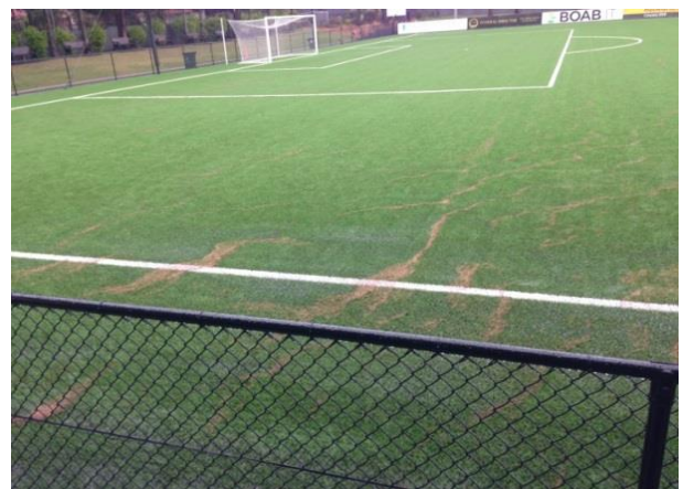
Photo 3: Organic infill displaced after rain, needs to be brushed to redistribute infill by using specialist machinery that can collect it and redistribute it accordingly. (Source: Smart Connection Consultancy)
